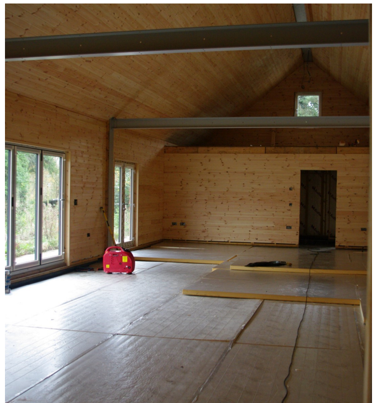
Inside cladding complete. Floor insulation going down. Next is the pipework for the underfloor heating.
