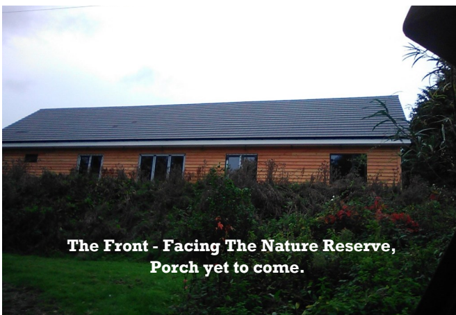
Wall cladding complete. Roof tiles in place. Double glazing installed. Gable end finished.
