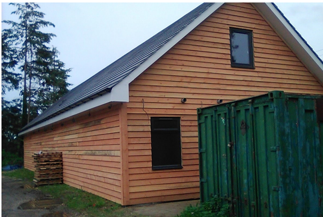
Wall cladding complete. Roof tiles in place. Double glazing installed. Gable end finished.
